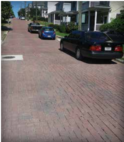
Figure 1. PICP is seeing increased use in municipal streets to reduce stormwater runoff, local flooding, storm pipe upsizing, and combined sewer overflows. These streets are in Atlanta, GA.
