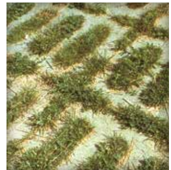
Figure 1. Grids first used in Germany in 1961 for overflow parking were building blocks placed in the ground. They emerged from the need to cool cities and decrease stormwater runoff.
