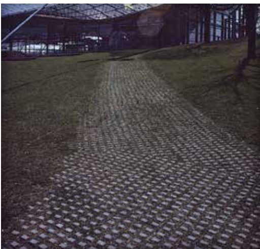
Figure 6. Service access lane
