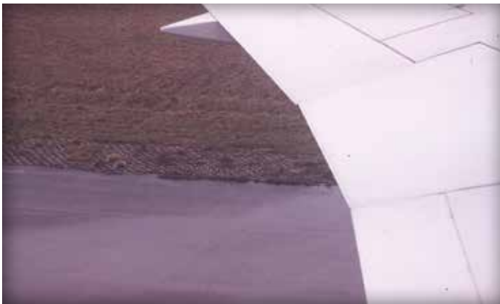
Figure 11. Airfield taxiway shoulder
