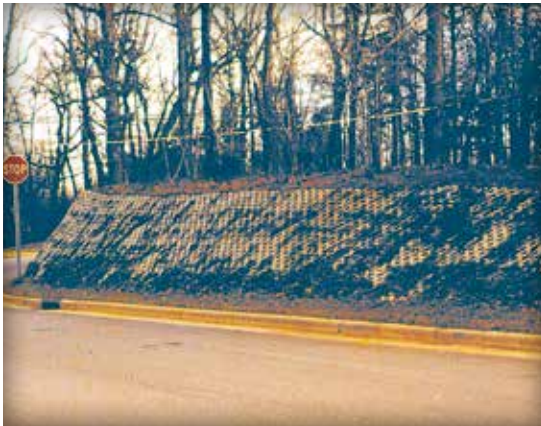
Figure 9. Embankment stabilization
