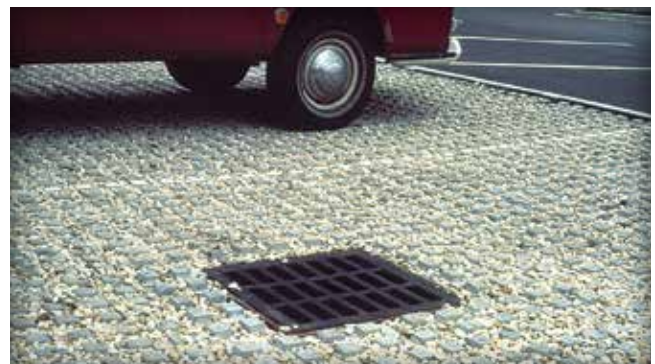
Figure 16. Concrete grids with aggregate in the openings
