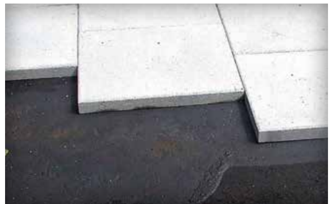
Figure 7. Sidewalk application illustrating the neoprene adhesive on an asphalt bedding layer under paving slabs
