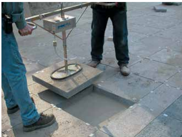
Figure 13. Two-person vacuum lift for paving slabs
