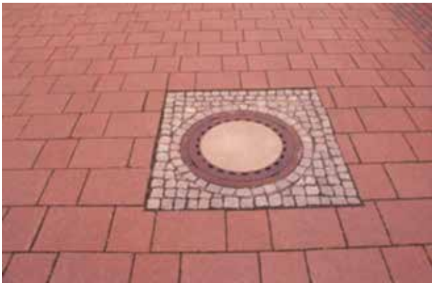
Figure 28. Filling the outside of a utility cover with mortar-set stone paving units
