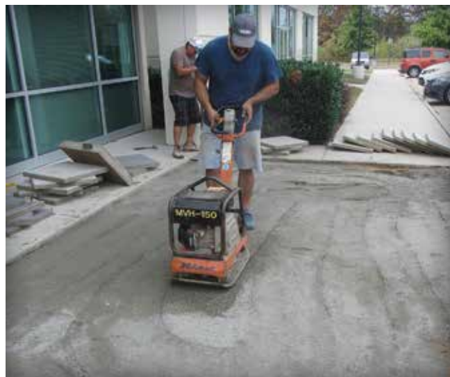
Figure 5. Precompacting the bedding sand
