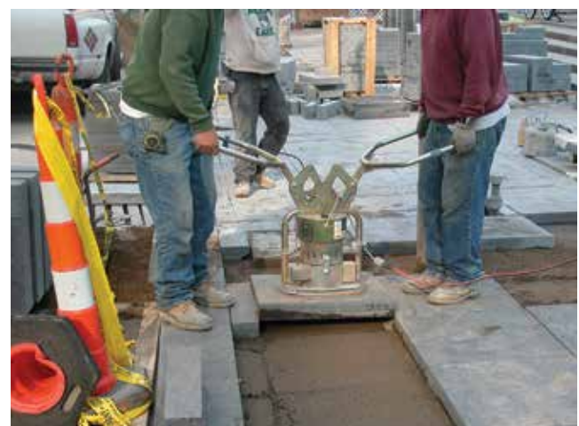
Figure 14. Two-person vacuum lift for larger paving slabs.
