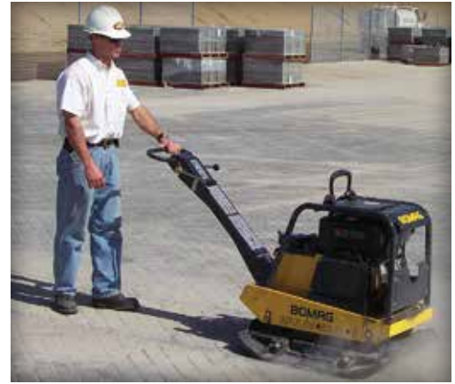
Figure 14. Second and final compaction of the pavers. The first compaction occurs after the pavers are placed (no sand in the joints). The second compaction works the sand on pavers into the joints. This process causes the pavers to interlock.
