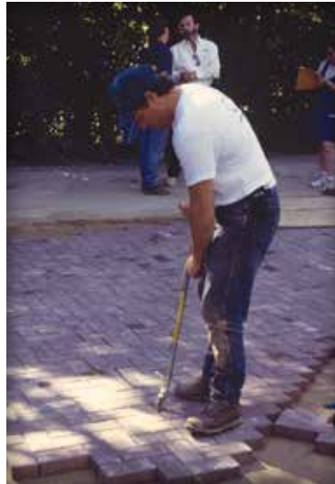
Figure 13. Adjusting joint spacing and alignment.
