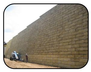
The water born staining process generally begins with a power wash, then a base coat, followed by one or two highlights. The highlights are "blended" into the blocks using a wet sponge to wipe the highlights off the block before they dry.
