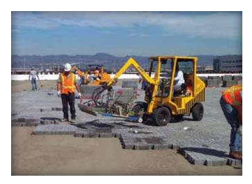
Figure 5. Motorized equipment with a hydraulic clamp.
