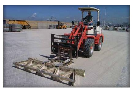
Figure 19. Broom attachments accelerate spreading and filling of joint sand.
