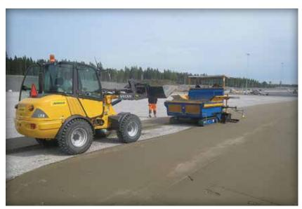
Figure 18. A screeding machine can evenly and rapidly spread bedding sand.
