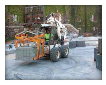
Figure 8. Clamps are an efficient method of moving cubes of pavers around the site, and can eliminate the need for wooden pallets.
