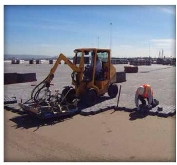
Figure 15. Spacing of cubes at the laying face is determined by how much area will be covered by each, as well as by the clearance required by the machine clamp. Orientation of the cubes follows the direction of paving.
