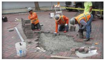
Figure 3. Once smoothed and joined with undisturbed materials at the opening perimeter, the bedding receives concrete pavers.
