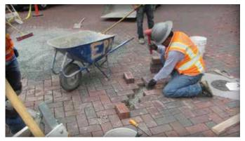
Figure 4. Reinstatment using the same pavers continues following the existing herringbone paving pattern.
