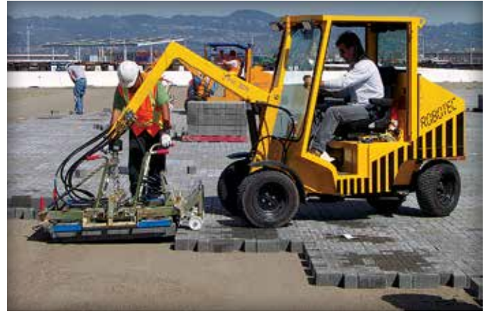
Figure 4. Hydraulic clamp picking up layer of pavers
