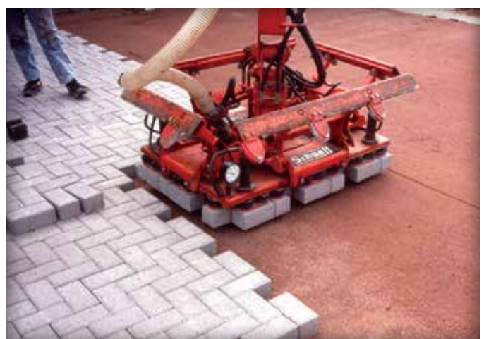
Figure 6. The vacuum head over the paver layer.
