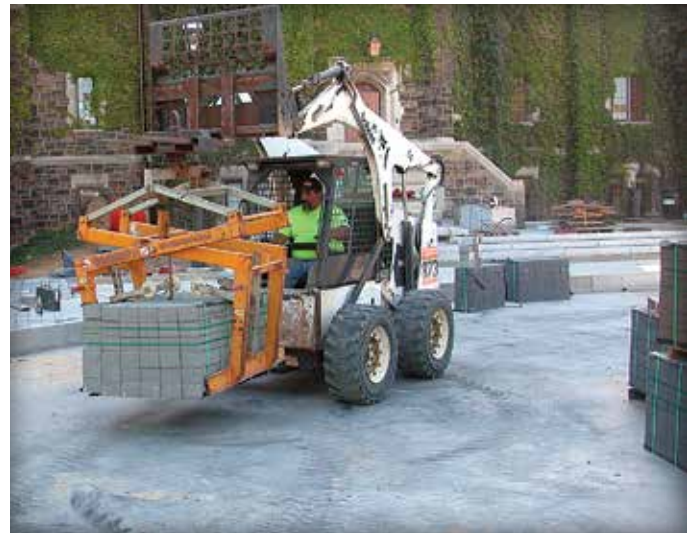
Figure 8. Clamps are an efficient method of moving cubes of pavers around the site, and can eliminate the need for wooden pallets.
