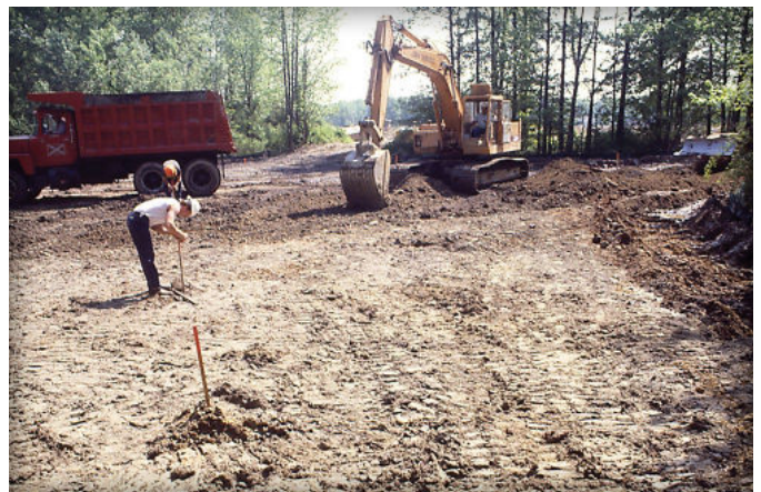
Figure 1. Excavation of the soil subgrade and placing grade stakes.
