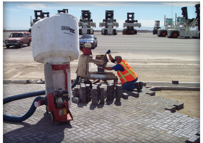
Figure 8. Saw cutting pavers.
