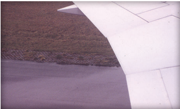
Figure 11. Airfield taxiway shoulder
