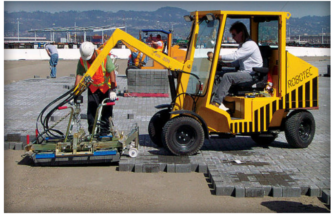
Figure 4. Hydraulic clamp picking up layer of pavers
