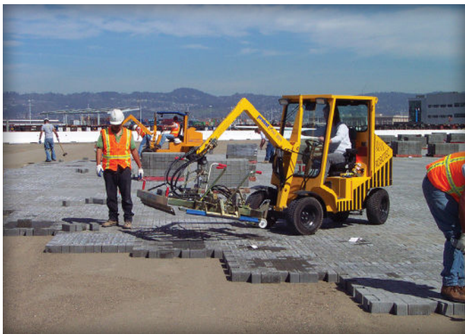
Figure 5. Motorized equipment with a hydraulic clamp.
