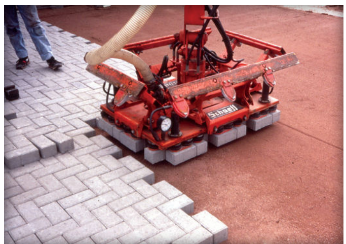
Figure 6. The vacuum head over the paver layer.
