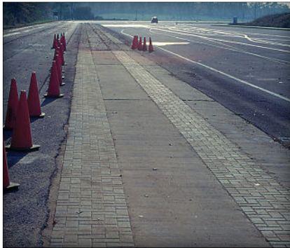
Figure 6. The test track section and concrete paver surface at The Pennsylvania Transportation Institute test facility.
