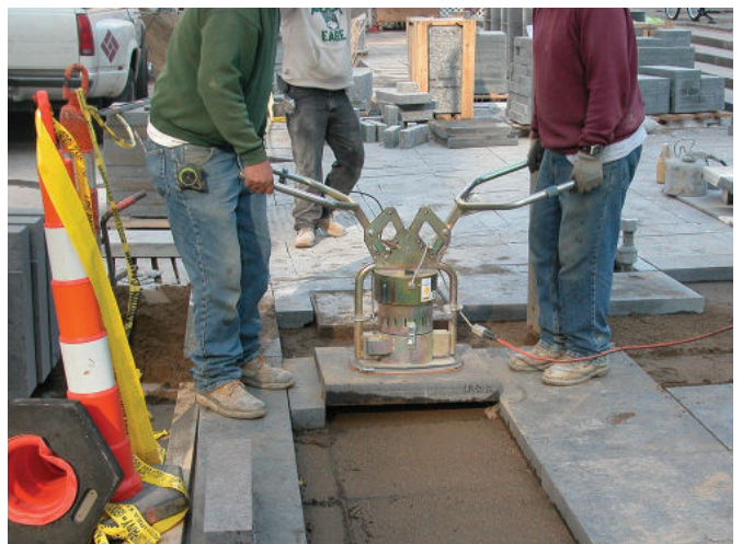
Figure 15. Two-person vacuum lift for larger paving slabs.
