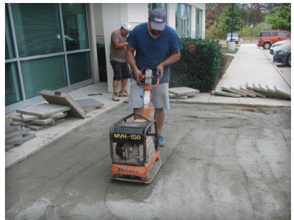
Figure 5. Precompacting the bedding sand
