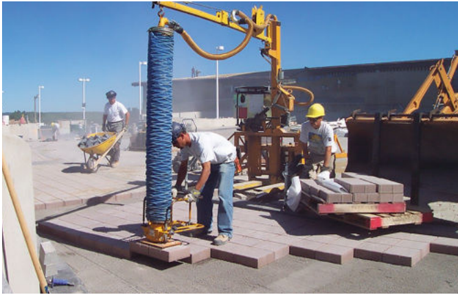
Figure 12. Self-contained vacuum lifter with boom
