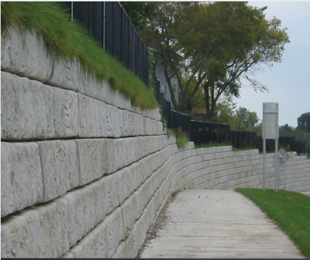
Gravity Retaining Walls
