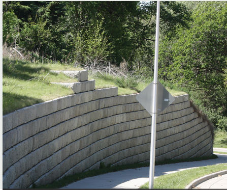
Reinforced Retaining Walls
