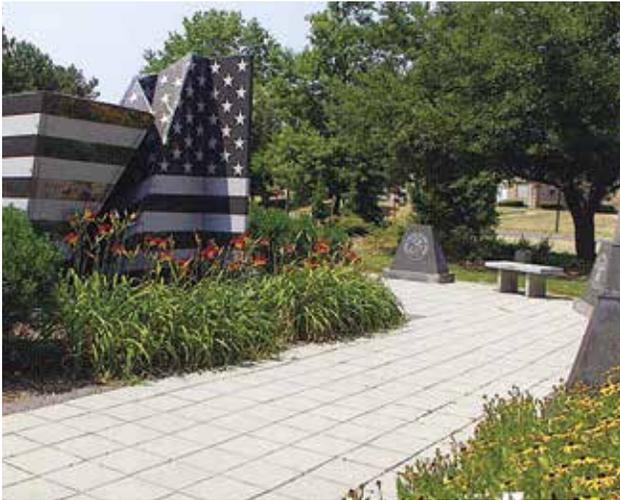
Figure 14. High SR paving slabs
