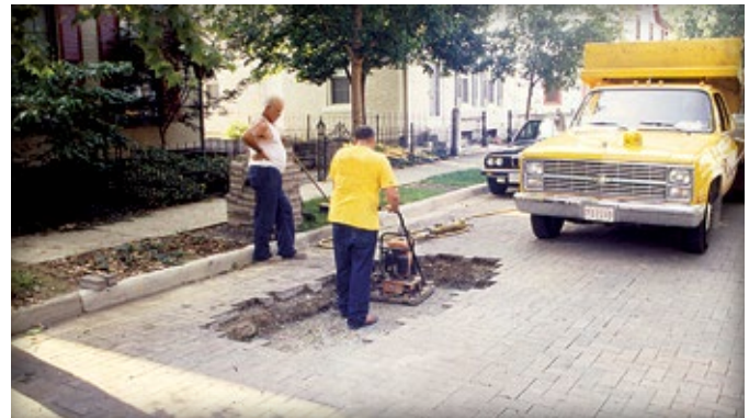
Figure 3. Compaction of the base
