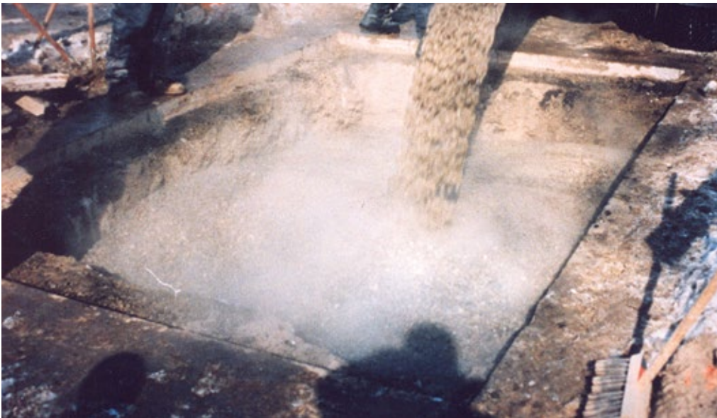
Figure 11. Low density concrete fill (unshrinkable fill) poured into a utility trench from a ready-mix concrete truck.
