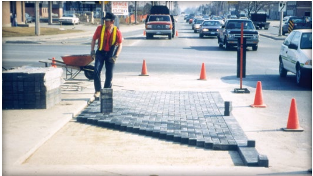
Figure 12. Pavers are laid in a 90 degree herringbone pattern between the border courses.
