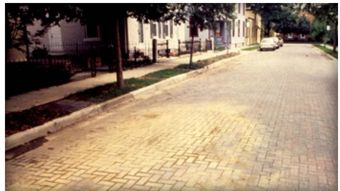
Figure 5. The final paver surface is continuous. There are no cuts or damage to the pavement.
