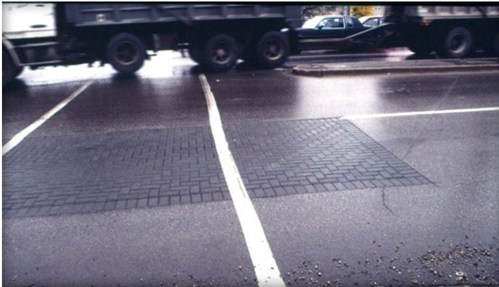
Figure 10. A patch of pavers in a heavily trafficked intersection in London, Ontario
