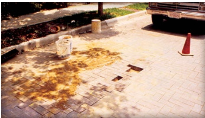
Figure 4. Reinstatement of the pavers, bedding and joint sand
