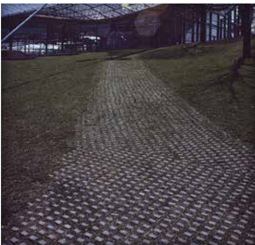
Figure 6. Service access lane
