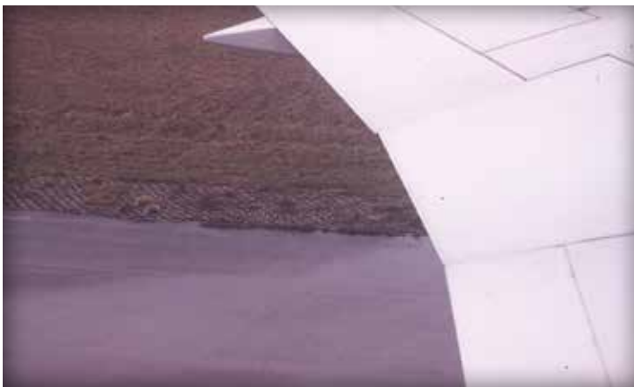
Figure 11. Airfield taxiway shoulder
